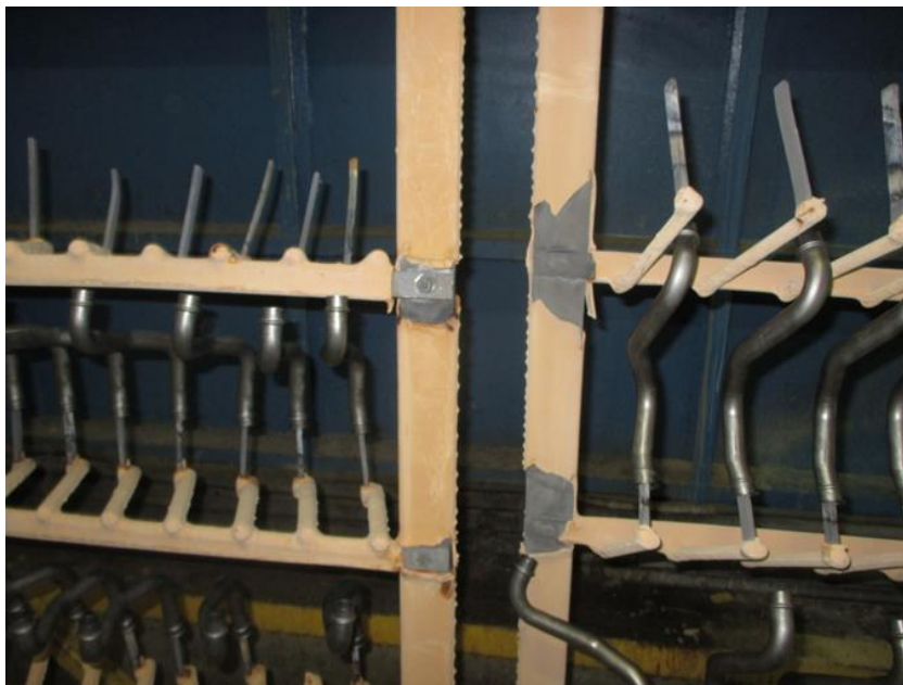
Figure 8. Rack Maintenance Issues
