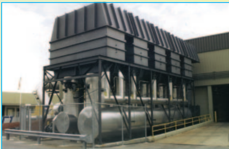
Chesapeake Finished Metals uses a custom RTO to destroy solvent-laden emissions efficiently for a wide range of loadings.
