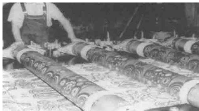
Figure 5—Printing with electroformed nickel screen cylinders (Photo courtesy of Nickelmesh AG, Rudolfstetten, Switzerland).
