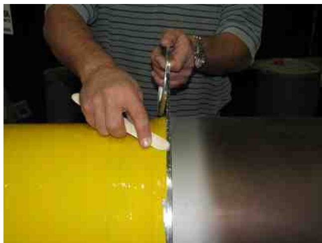
Figure 1 - Application of a metallic tape.
